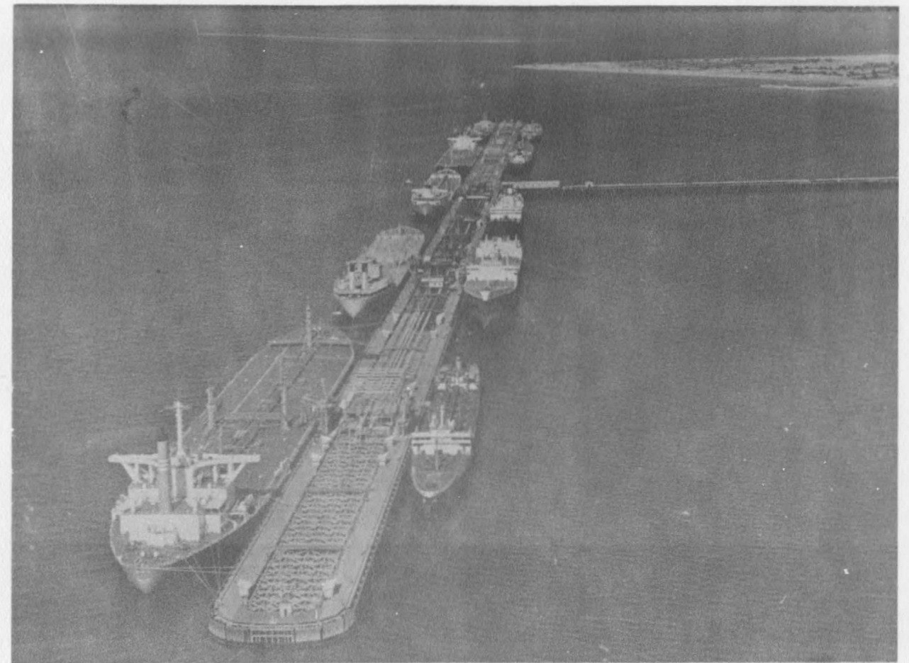
Kharg Island export terminal capable of berthing 10 oil tankers of up to 500,000 tons.
