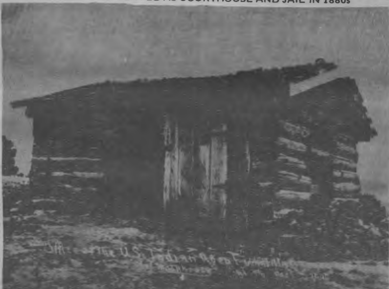
BIA BUILDING SERVED AS COURTHOUSE AND JAIL IN 1880S
