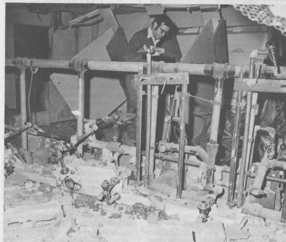
Workmen check the extensive damage, repair cracked water pipes.
