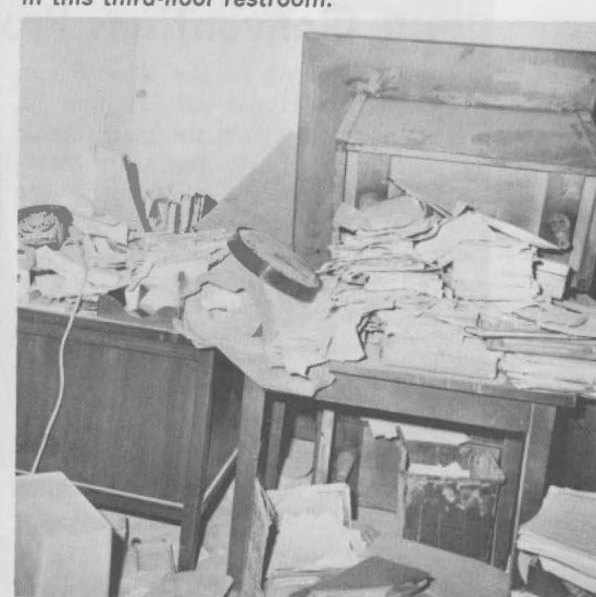
One of the 20 offices which were heavily damaged by the bomb.
