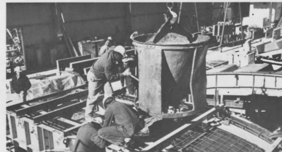
Casting concrete coffer in Hyattsville for Dupont Circle station.
