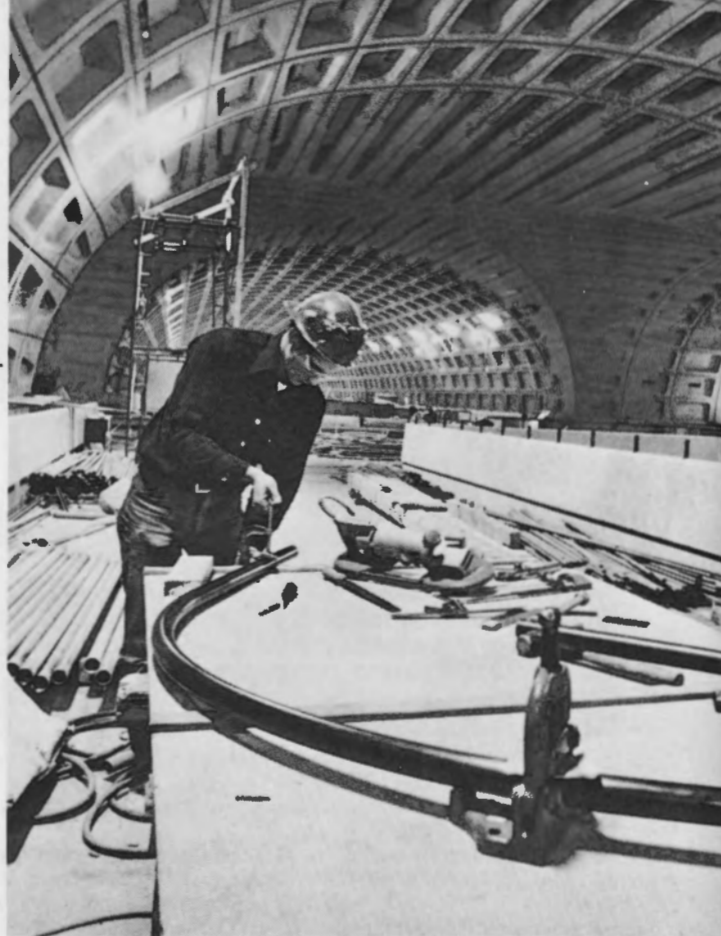
Workman shapes bronze handrail for Metro Center station.
