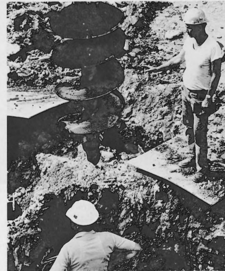
While finishing touches are added elsewhere, construction starts at other sites.
