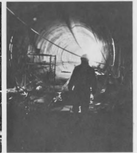
Pentagon station passageway (right) will connect underground to bus platforms. A concrete-lined tunnel.
