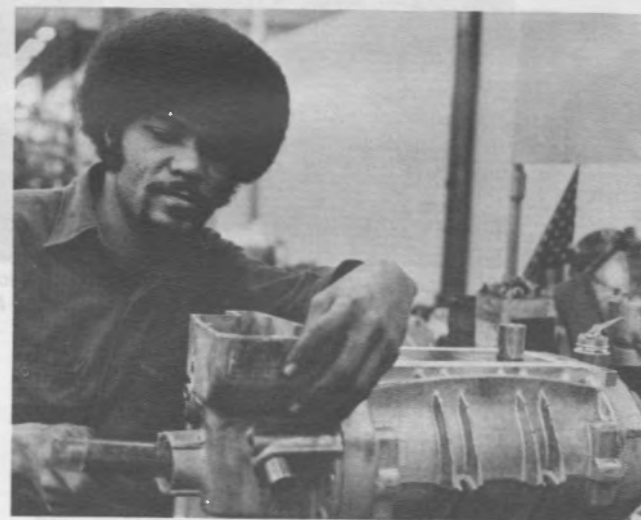
Mike Holley, mechanic, overhauls an engine blower in the small units shop of the Bladensburg bus shop. When he is finished, the blower will be stored in a huge supply room to be used, later, as a replacement part.
