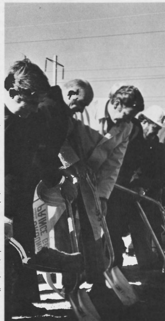
First Maryland ground is turned for Silver Spring station.
