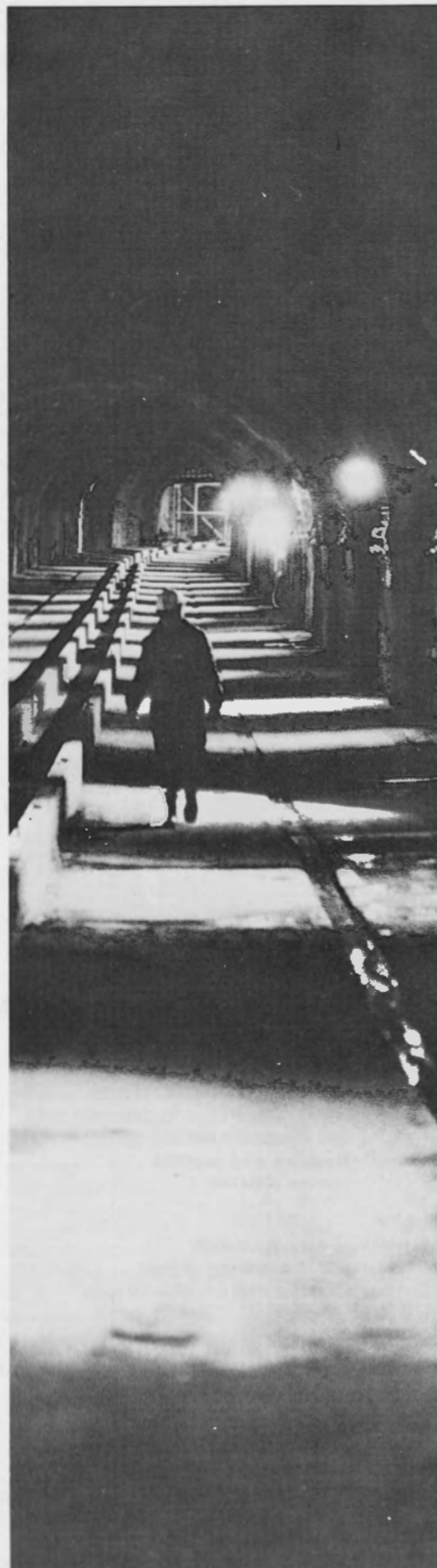
Rock tunnel under Connecticut Avenue awaits first rails.
