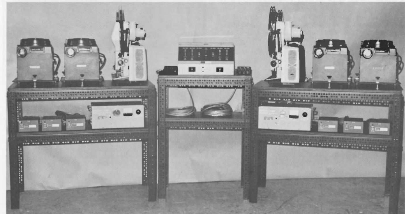
Dual Front Projection System for use as dual system in a large auditorium or as two individual systems in a split auditorium.
