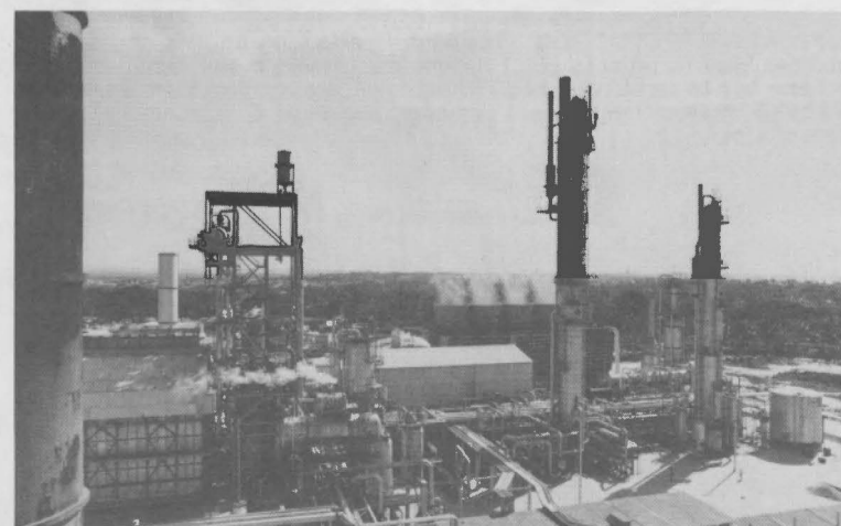
ONSTREAM IN MEXICO: The first Kellogg-designed ammonia plant in Mexico has gone onstream at Cosoleacaque. The 1000-ton-a-day facility went into full production within 12 days of first feed. Kellogg has contracts for design and engineering of three more plants for Pemex—two 1500-ton-a-day units to be built at Cosoleacaque and one 1000-ton-a-day facility to be constructed at Salamanca.
