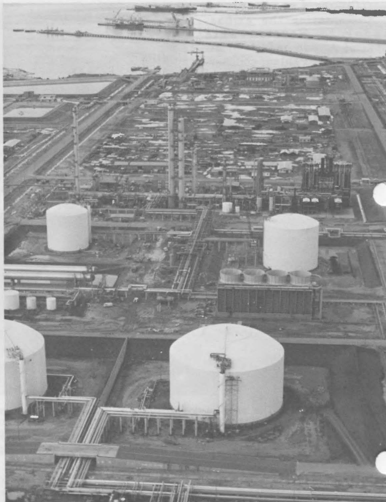
EL TABLAZO SCENE: A view from the air at El Tablazo, Venezuela, shows the Kellogg-built ethylene/olefins unit. The two long piers in the background also were Kellogg's responsibility. The nearest is for liquids handling; the second for solids.
