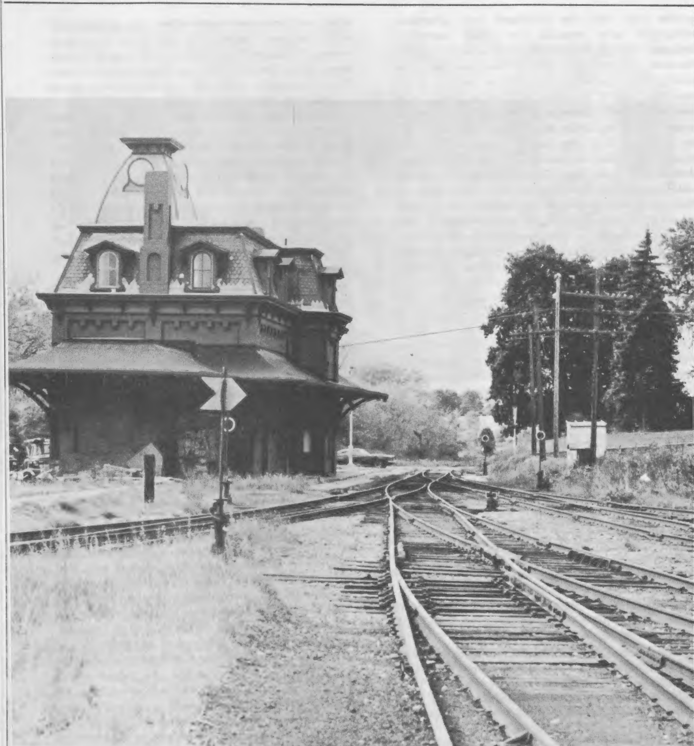
The exterior of the North Bennington Railroad Station looks much the same as it always has, but the interior is being currently remodeled to house offices.
