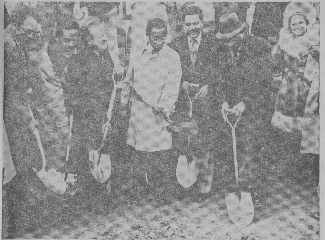
NEW TOWN IN THE MAKING — Dignitaries break the ground for the construction of a "city within a city" on the territory at the northeast edge of Washington. (L to R) D.C. Councilman William Spaulding; Emanuel Lipscomb, chairman of the Mayor's Advisory Committee on Fort Lin-
