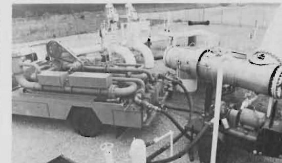
Master Meter Unit
